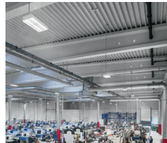
Replacing indoor lighting with steered LED-lighting
